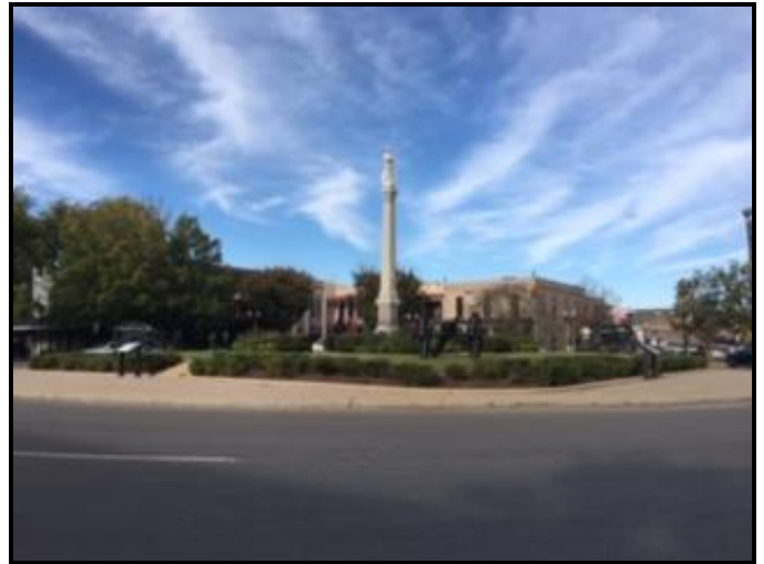
The two markers on the island are installed on the street-level sidewalk near the steps onto the upper level. Visitors will face the Monument as they view the markers.
