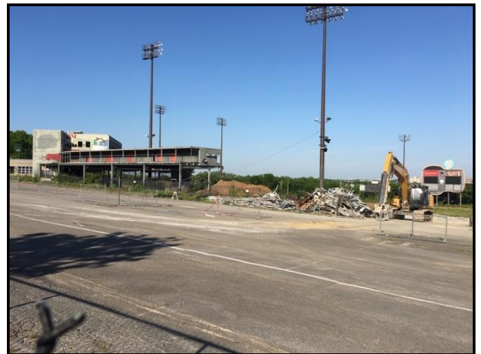
Demolition equipment begins removing the seating area behind first base line
