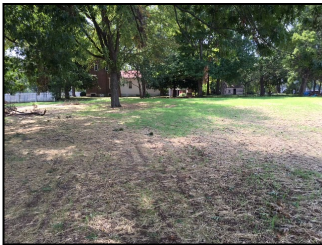
The old Franklin High School site looking south to the Carter House shows the new grading and the grass starting to cover it.
