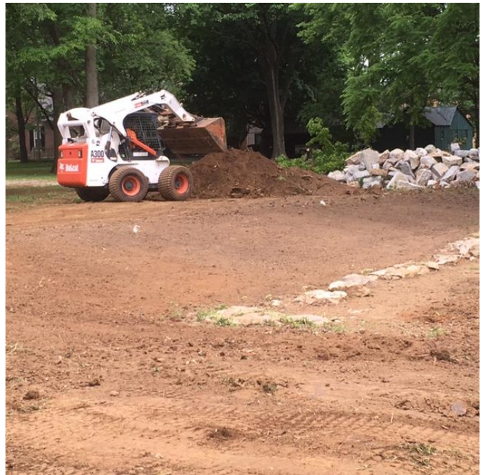
Park employees smooth and dress the grade around the Cotton Gin foundation in right foreground
