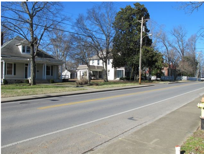
The two Lovell houses are located just south of the Carter House (red brick house on right)
