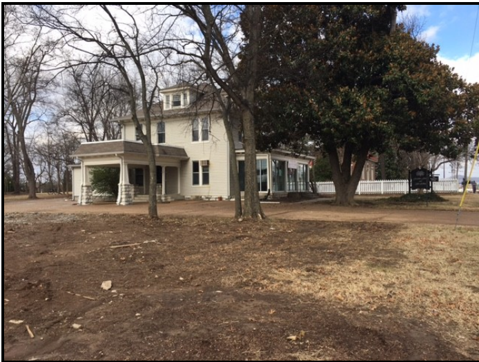
The Lovell house (flower shop) will be dismantled and removed in January. The Carter House is beyond the white fence in the background to the right.
