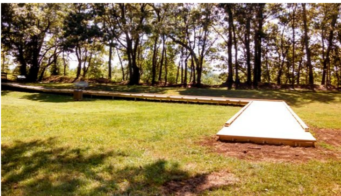
Work continues on the new walkways
